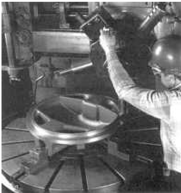
Cast domed disc being machined.
