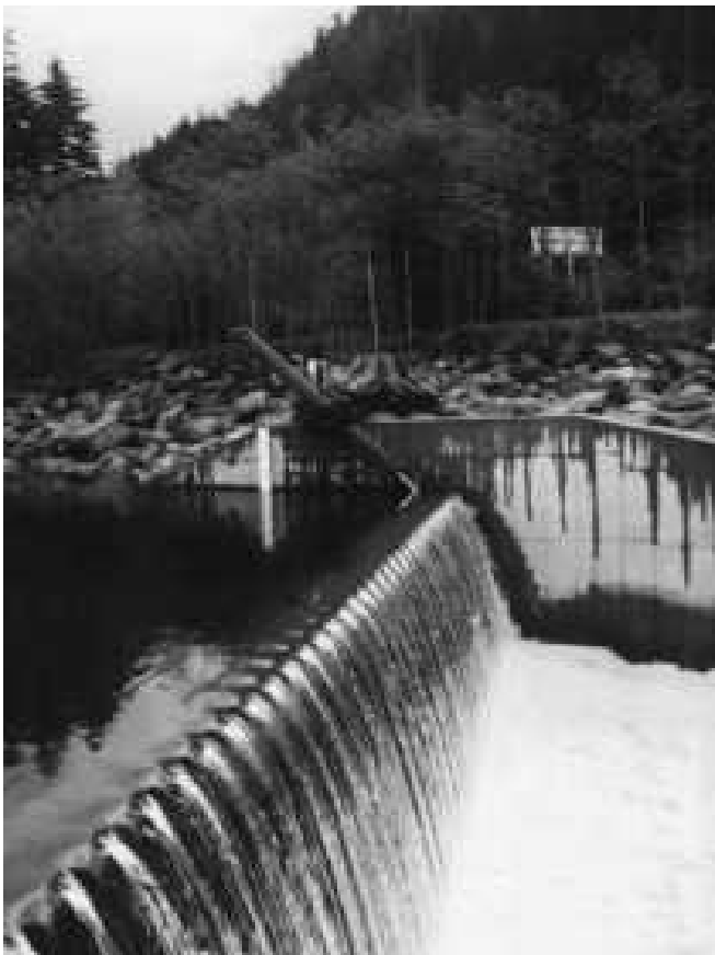
A 65' x 10' high crest gate on the Snoqualmie River in North Bend, Washington. Hydraulic system consists of two top-mounted hydraulic cylinders (2000 psi).
