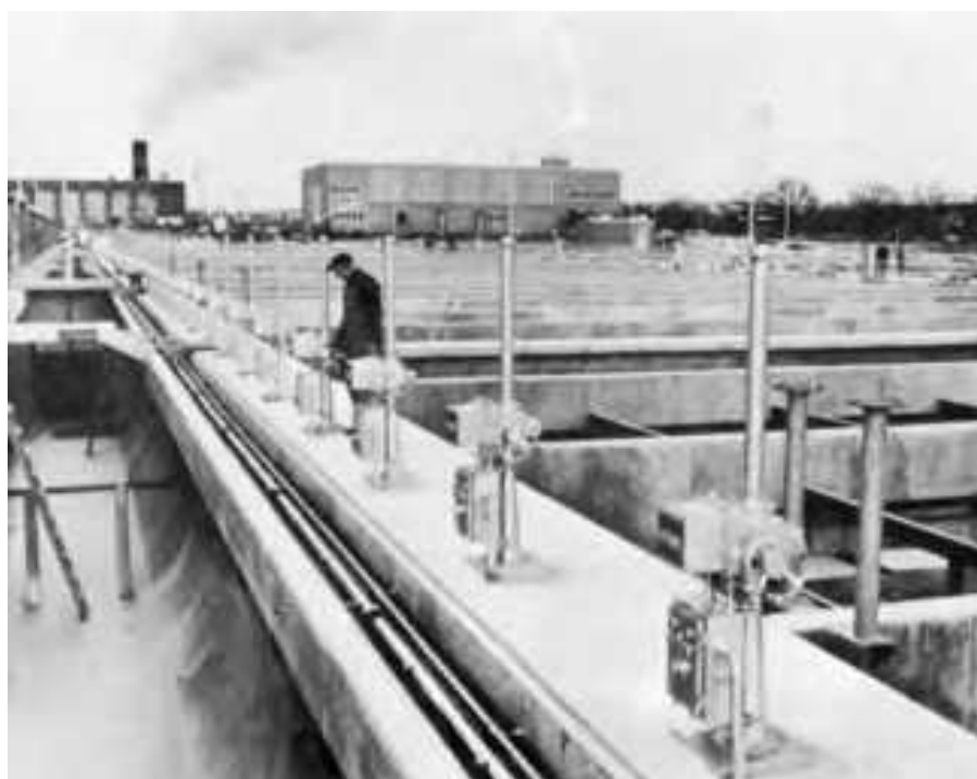
Limitorque and E.I.M. electrically operated floor stands used in typical treatment plants.
